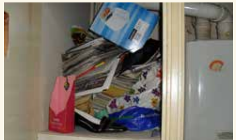
✗ Not acceptable standards
